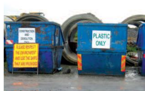
Figure 5: Example of Good Waste Segregation (Source: National Roads Authority)
